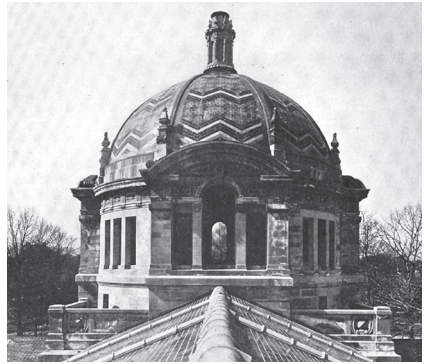
Guastavino dome. Elephant House, Bronx Zoo. C. H. Hughes. (1909). "Interesting Examples of the Use of Burnt Clay in Architecture", The Brickbuilder , Vol. 18, No. 8, pp. 158-159.
